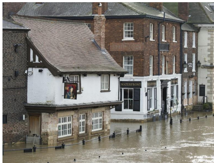
Severe flooding. Source: © Don Lodge/Unsplash, 2024.
